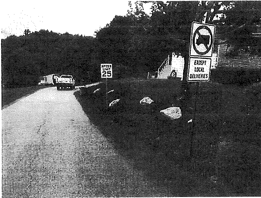
Replaced Speed Limit 25 Sign with New Sign (Near Finleyville Elrama Road – Heading South)
